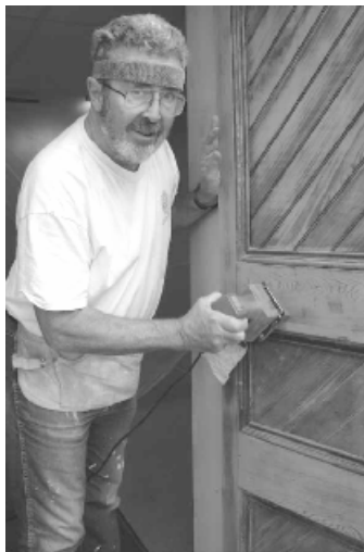
Ron Cook sands a door in preparation for painting at St. Georges's
